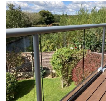
Glass Panels for the balcony.
