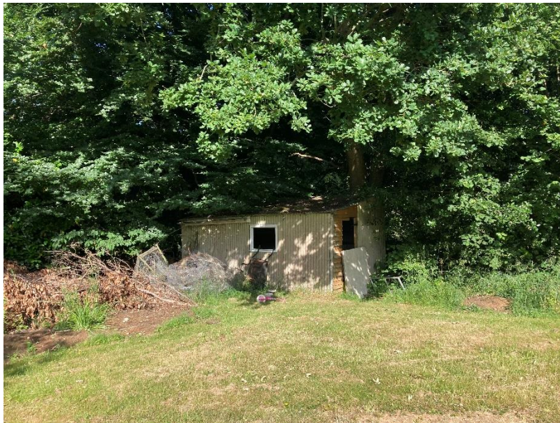
Photograph 8: View of low potential building in north-east corner of Application Site
