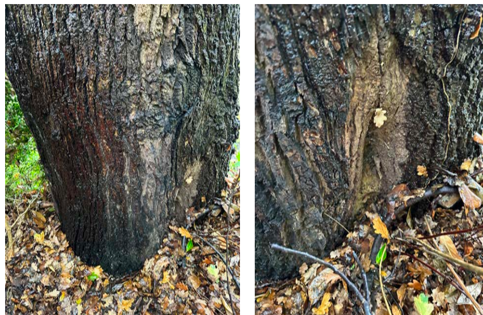
Figure 4a & 4b: Bark damage to North East of the main trunk
