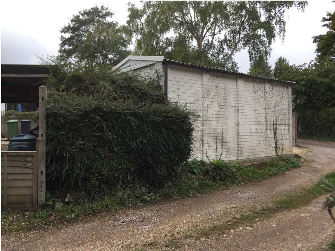
REAR VIEW OF GARAGE FROM THE PRIVATE ACCESS ROAD
