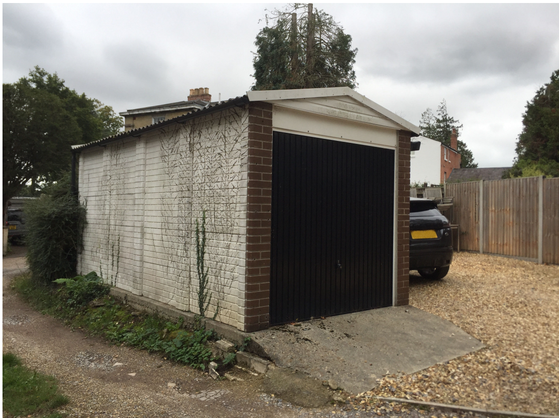
VIEW OF GARAGE FROM THE PRIVATE ACCESS ROAD
