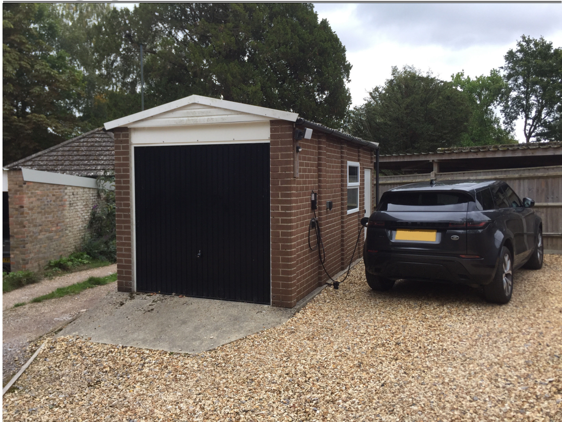
GARAGE WITH ADJOINING CAR PARKING SPACES
