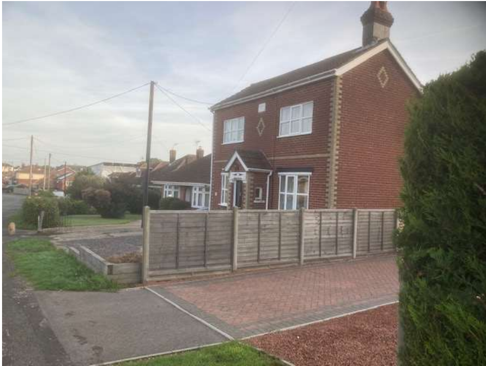
Fig.4 – Photo looking towards the side elevation of the 2-storey house at 31 Hobb Lane with the application site in the background (2 doors down).
