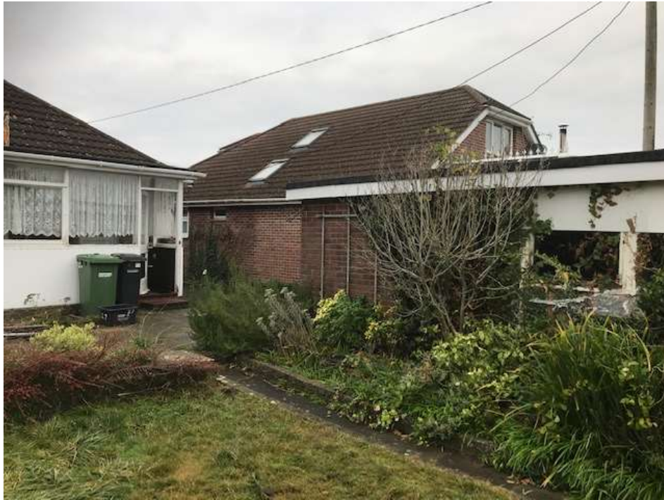
Fig.2 – View from the rear garden of 27 Hobb Lane showing the existing garage and rear elevation of the bungalow (left).
