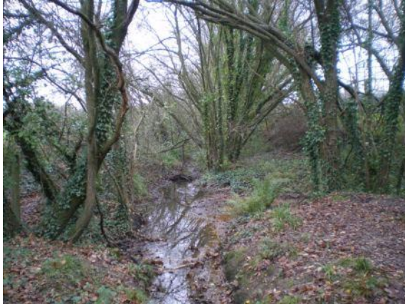
Photo 1. Culvert with woodland on the banks - area to be removed. (Taken 09/12/20)
