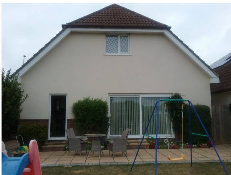
View at rear of building
