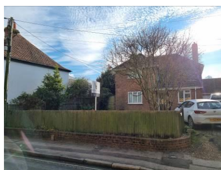
Ferndale and Church Cottage to east
