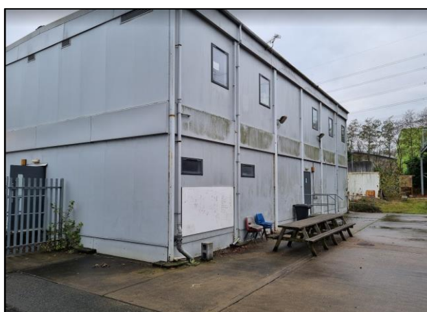
Photo 5 Existing two-storey modular building (Wessex House).
