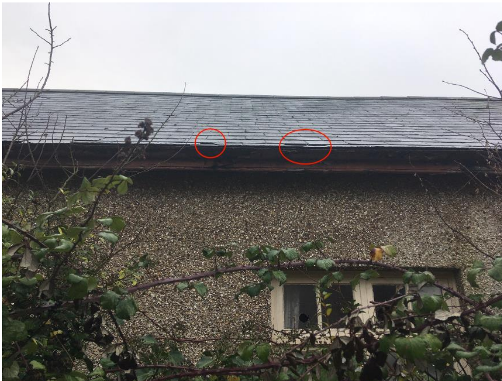
Figure 3: Slate tile roof with potential gaps for bats.
