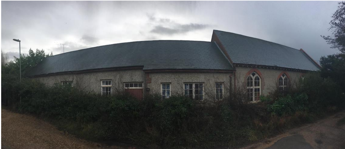
Figure 2: Church as viewed from the north
