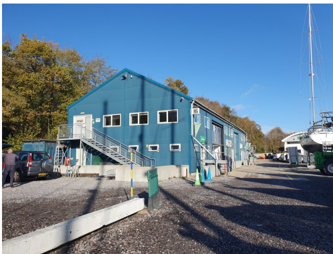
SW end gable.
