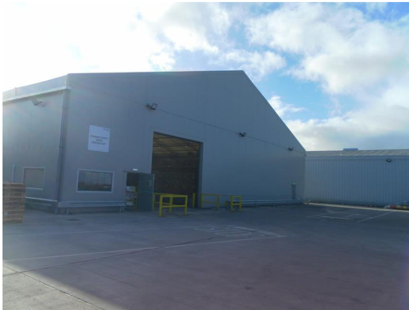
.North elevation of existing Spaciotempo storage building
