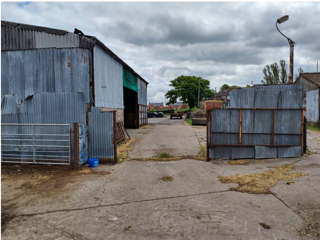
Plate 4 – View east across the site
