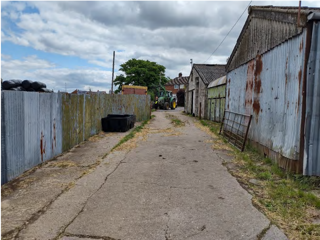
Plate 1 – View east across the site
