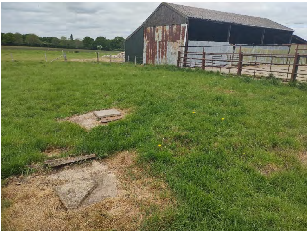
Plate 14 – Current septic tank in south of the site
