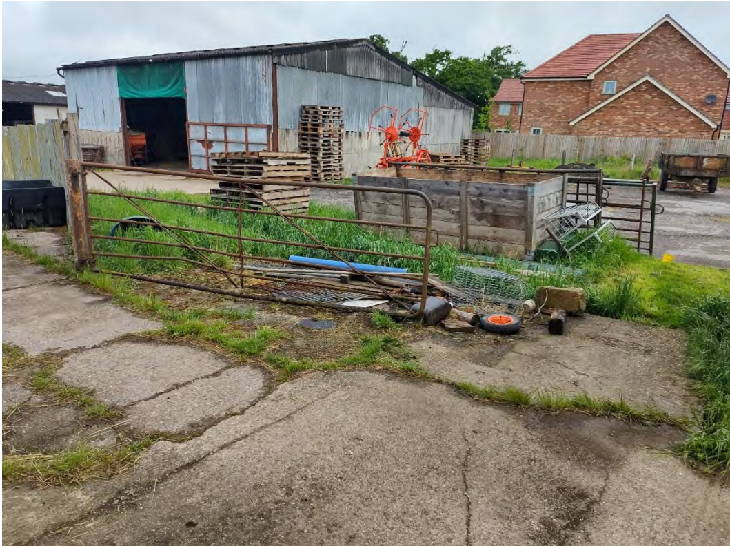
Plate 13 – Defunct septic tank location
