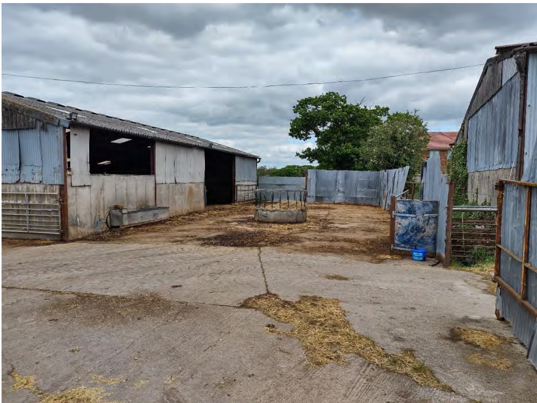
Plate 2 – View north across the site
