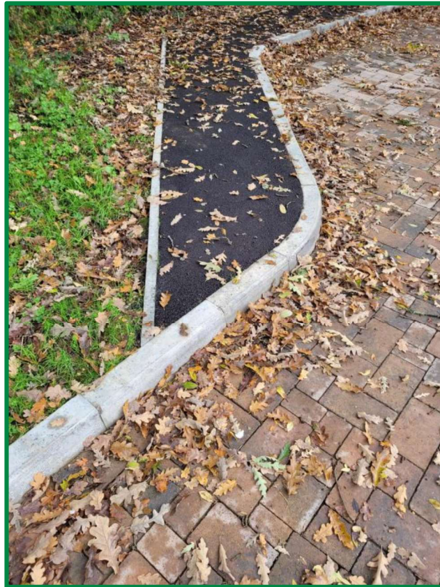
Photo 32 – Full Height Kerbs Installed
