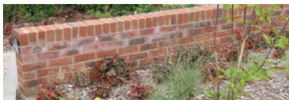
Low Brick wall
