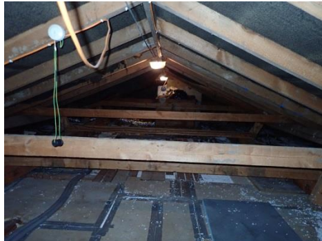
Main loft space
