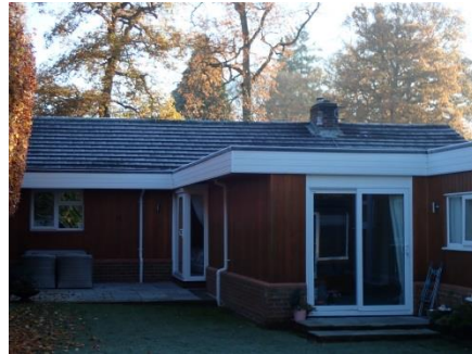
Rear/western elevation (with flat roofed extension)
