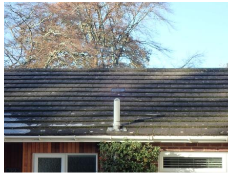
Tightly-fitting roof tiles throughout
