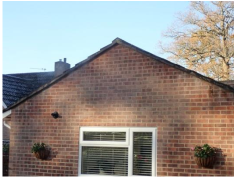
Front gable showing sealed verges
