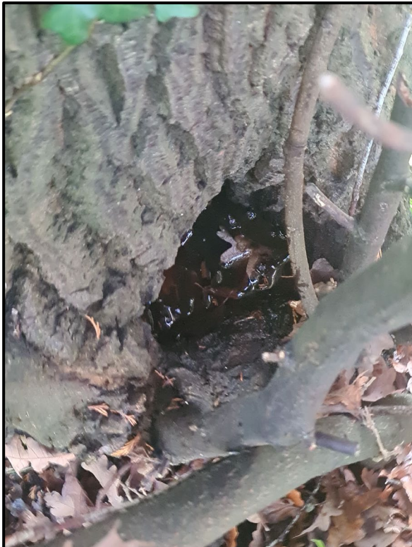
Photograph Two – Cavity at base of T2
