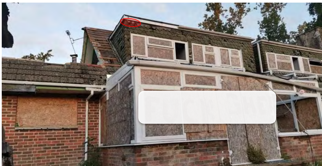
Figure 27. Approximate locations of 2 x Common Pipistrelle emergence (Red dot) on the north west facing aspect during the first survey.
