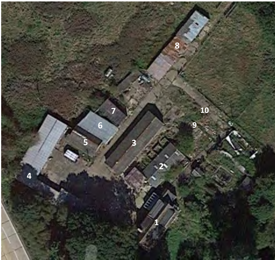
Figure 14. One dwelling and 9 outbuildings on site with their associated numbers.
