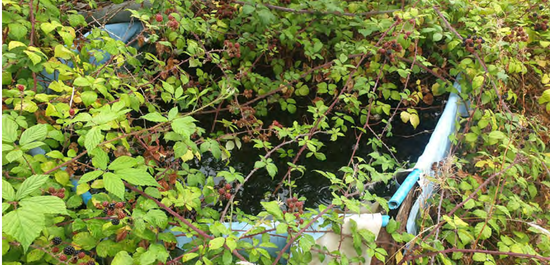
Figure 12. New pond identified to the south east of the dwelling (August 2022).
