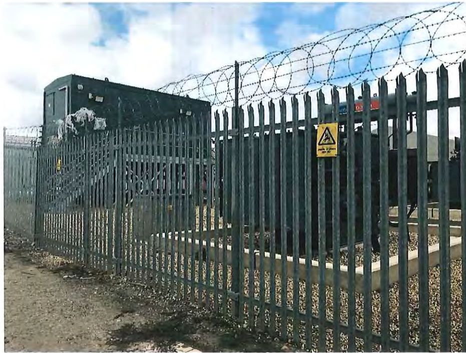
Photo 3 The electrical substation adjacent to the site
