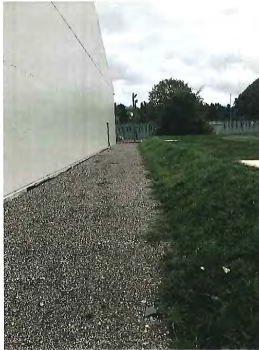
Photo 1 Looking east along the southern side of Unit 1
