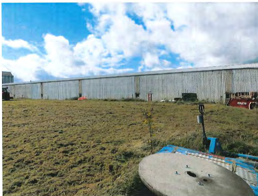
Photo 4. View of the Unit 1 area from the north-east. Photograph taken 01/10/21
