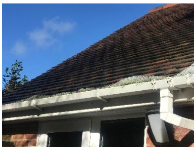
Rear of the garage roof on south western side of the house.
