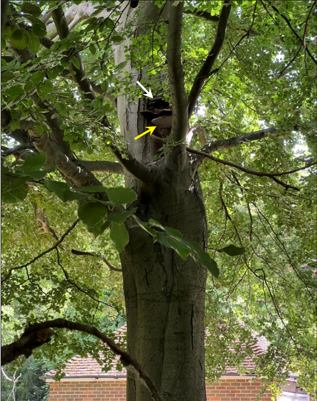
Figure 1: View of the multiple Ganoderma sp fungal brackets on the trunk of T13, showing the newest, largest, and most active bracket with the white underside on the lower side of the cluster (yellow arrow), and the older browner decaying brackets on the upper side of the cluster (white arrow).
