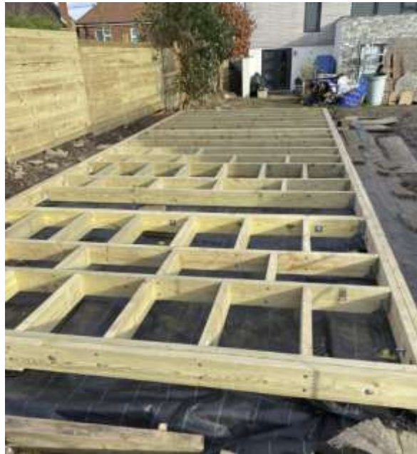
Fig 10. Wooden Foundation Frame – SH1
