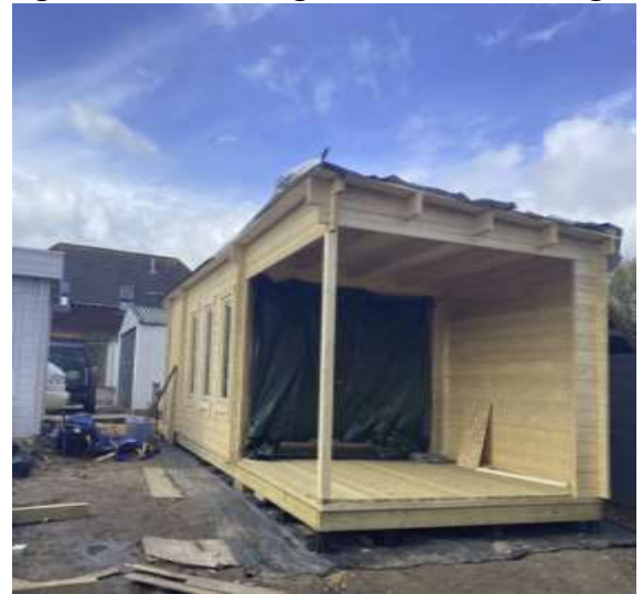
Fig 13 – SH1 Decking Area – Current Height
