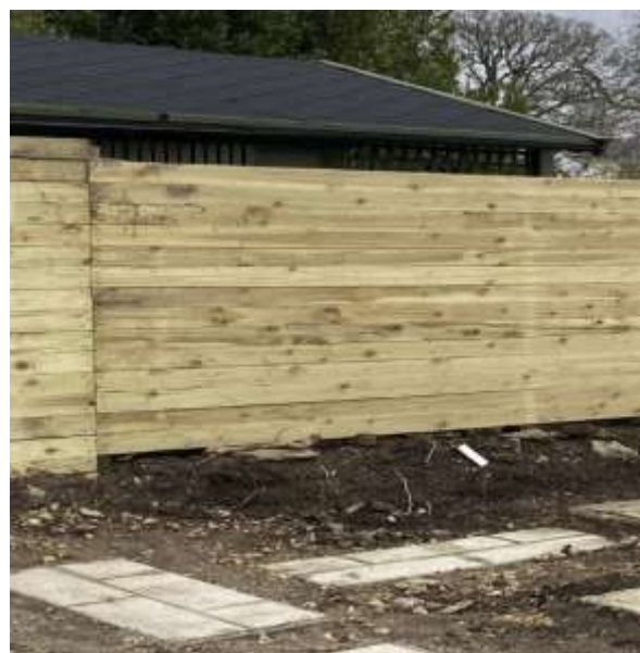
Fig 9. Reduced Ground Height After Levelling
