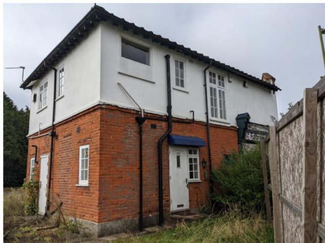
Picture 2: Building B1- Northern aspect.
