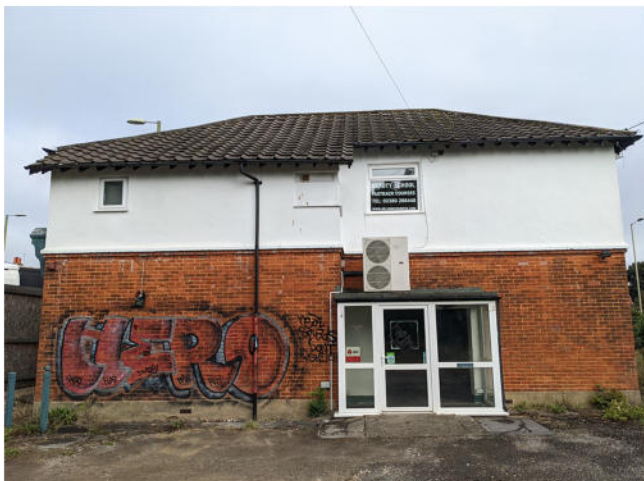
Picture 1: Building B1 - Southern aspect.
