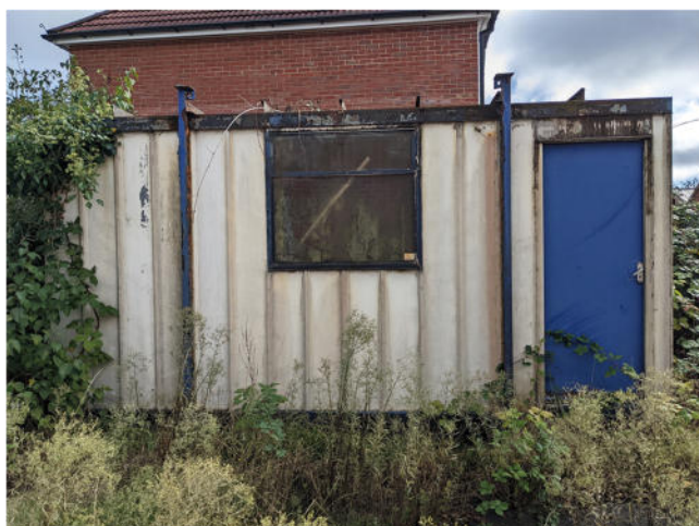
Picture 6: Building B2 on eastern boundary of the site.
