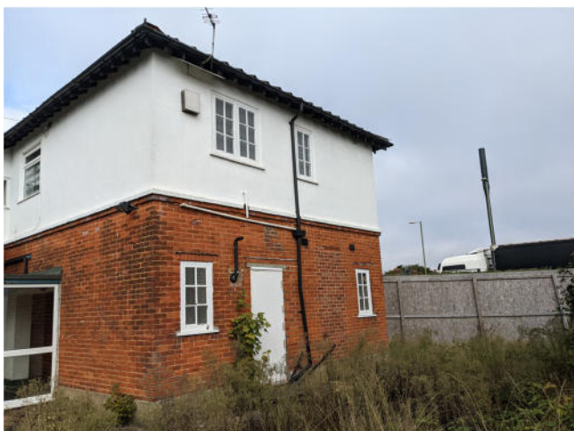
Picture 3: Building B1 - Eastern aspect.
