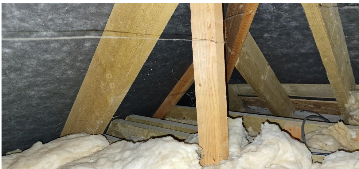
Picture 5: Showing the roof spaces and the breather membrane
