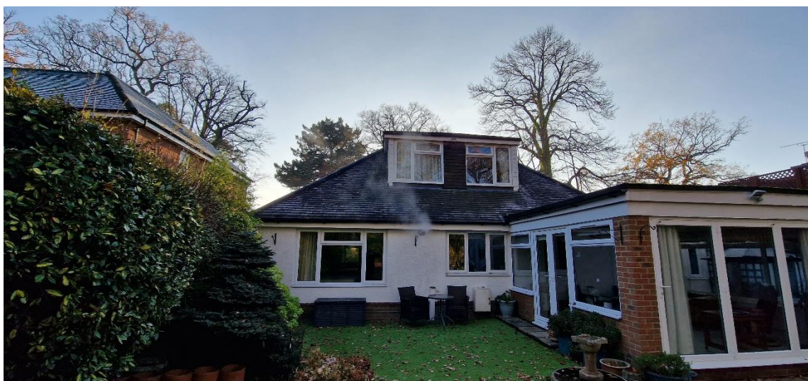
Picture 2: Showing the rear elevation.
