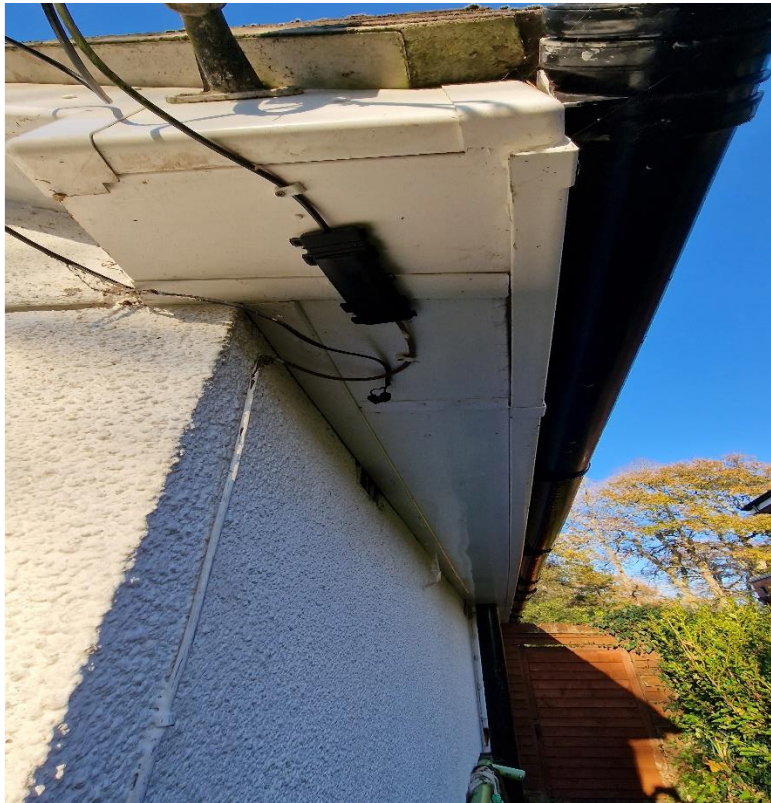
Picture 3: Showing the UPVC soffits and eaves
