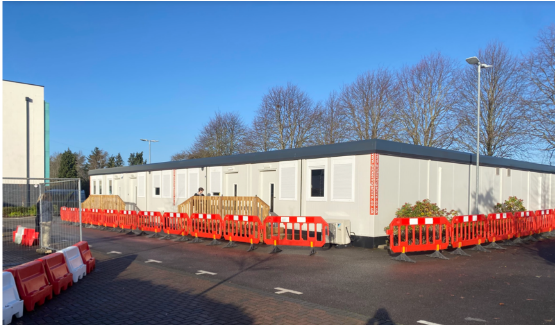
Figure 7. View of the southern and eastern elevation of the temporary building on site (taken November, 2022).
