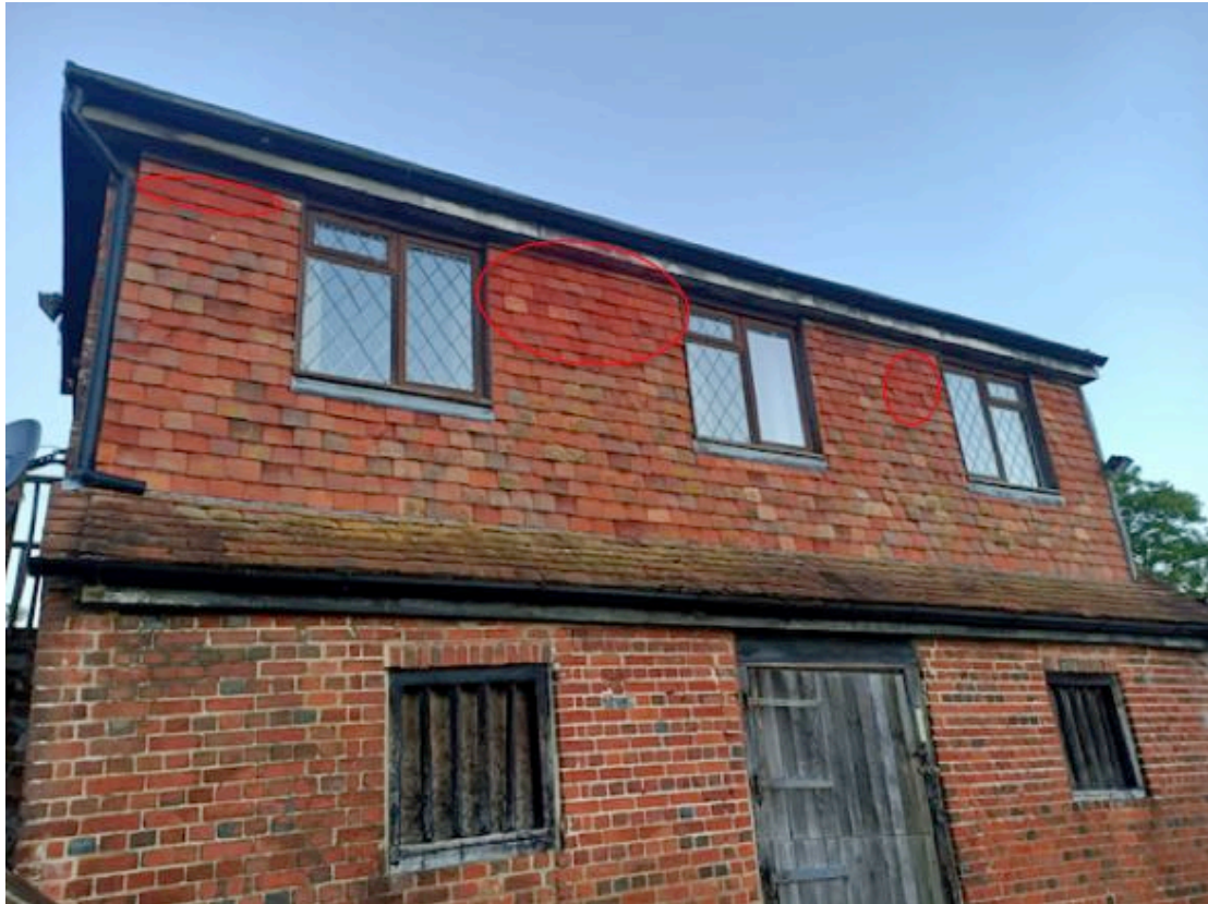
Figure 16. Approximate locations of the Common Pipistrelle roosts on building D (Red circle) during all surveys.
