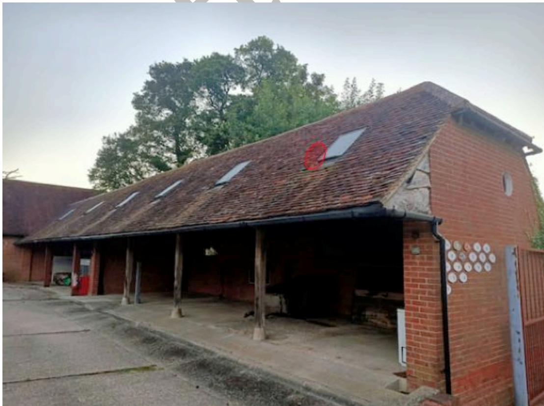
Figure 17. Approximate locations of the Common Pipistrelle roosts on building A (Red circle) during the first survey.
