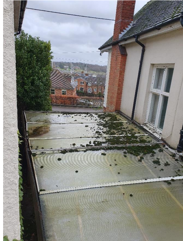
Figure 10: Boundary line between 13 and 15 Satchell Lane. The carport boundary sits 50cm inside the boundary of 15 Satchell Lane.
