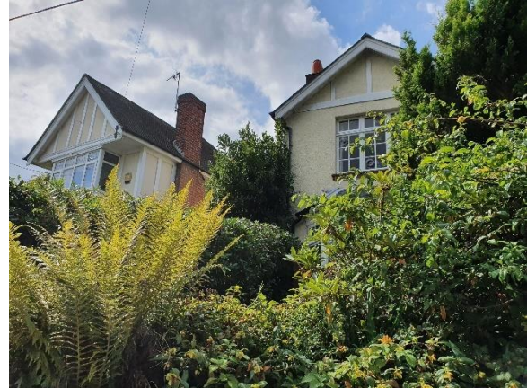
Figure 2: The proposed ground floor extension with terrace, and the third storey extension is out of character with the street scene. There are no other three storey properties between 1 and 21 Satchell Lane and the exterior design is also out of character in comparison with the adjacent properties.
