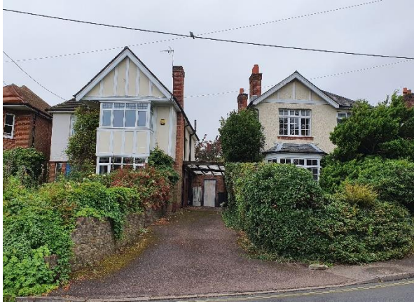
Figure 1: The proposed excavation to road level (removal of 150 tonnes of soil) for the enlargement of parking area, and the north elevation ground floor extension adjacent to subsidence at 15 Satchell Lane will impact on land stability. Also, the ground floor extension (east elevation), 1m beyond the footprint, will deny 11 Satchell Lane amenity (privacy, noise).
