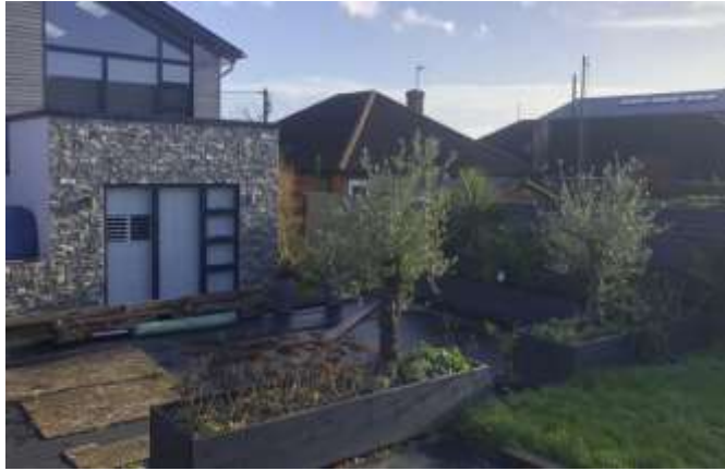
Fig 6 - View SE from SH1 decking to No 7
