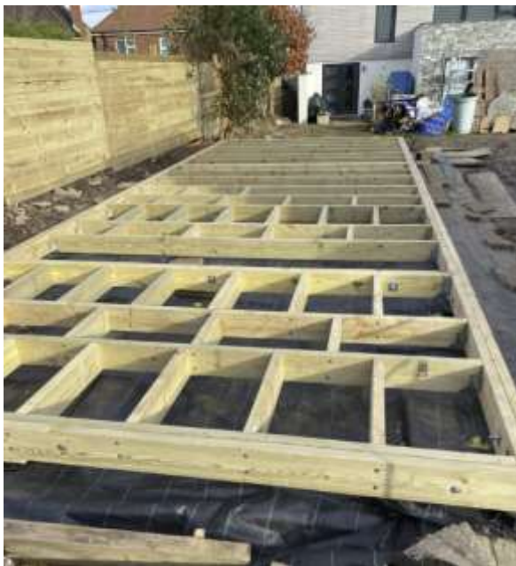
Fig 10. Wooden Foundation Frame – SH1
