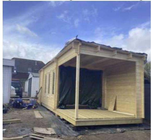
Fig 13 – SH1 Decking Area – Current Height
