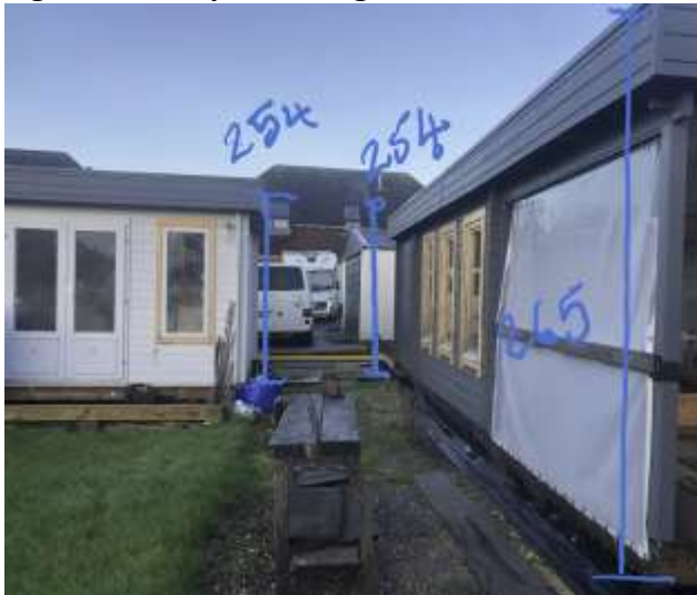
Fig 12 – Anticipated Heights at final Ground Level
