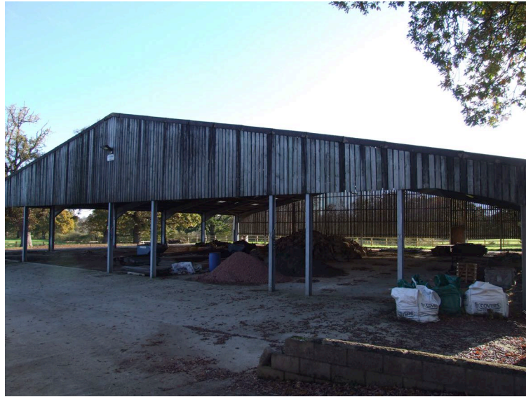
View from Barn B obstructed by Barn F
