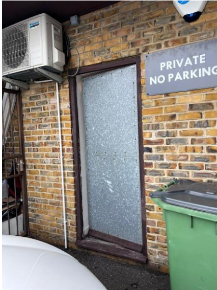
Fire Exit & Access to Back of Shop
