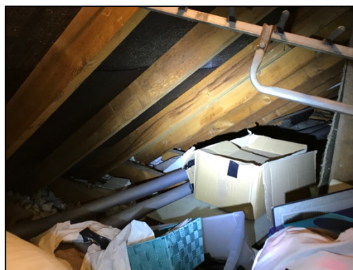
Figure 4 – roof void with bitumen lining and stored items
