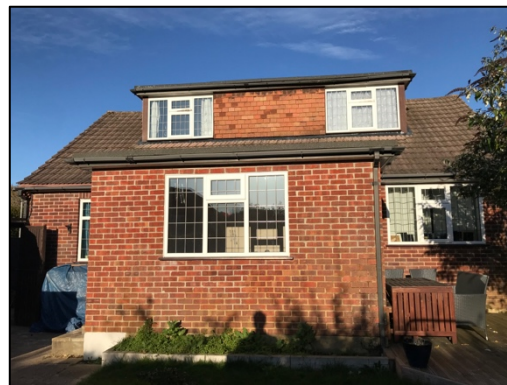
Figure 2 – south-western elevation with extension and dormer windows
