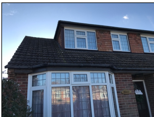
Figure 3 – north-eastern elevation with bay window and dormer windows
