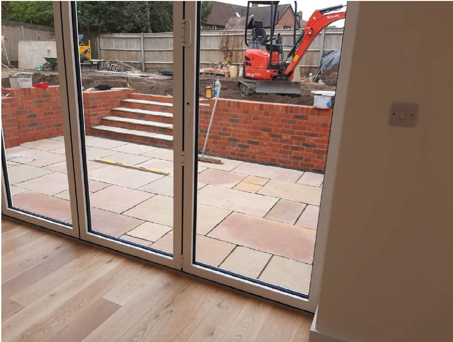
19336 The Malthouse: Site Works Photograph – View SW from House Interior
