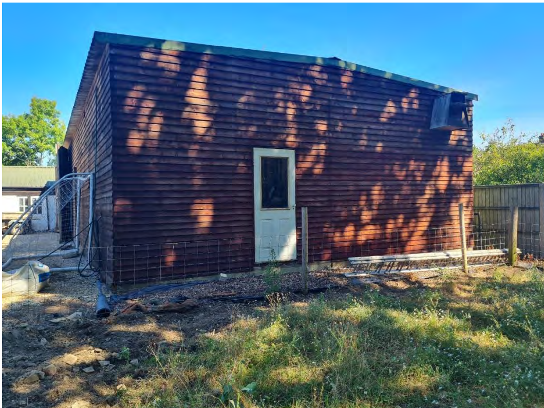
Side elevation of Building 2
