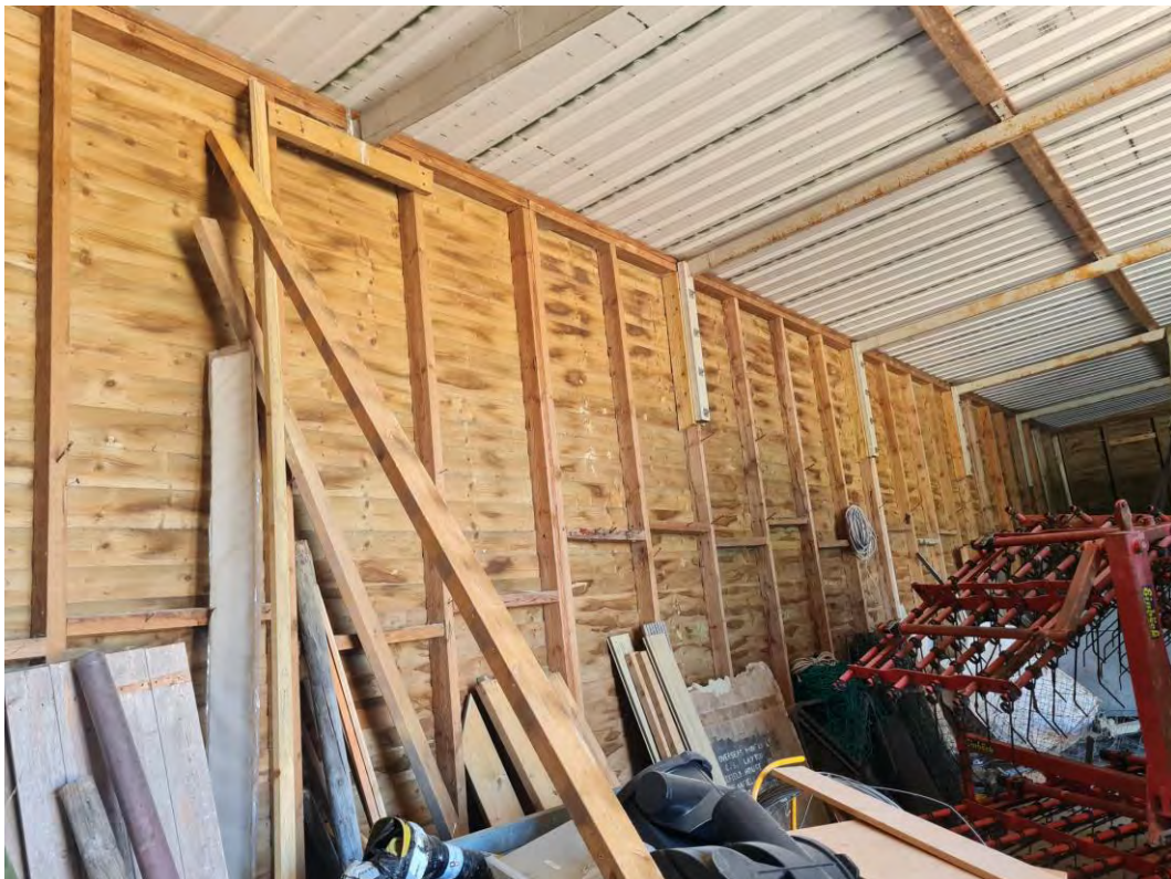
Internal view of Building 2 including bailer
