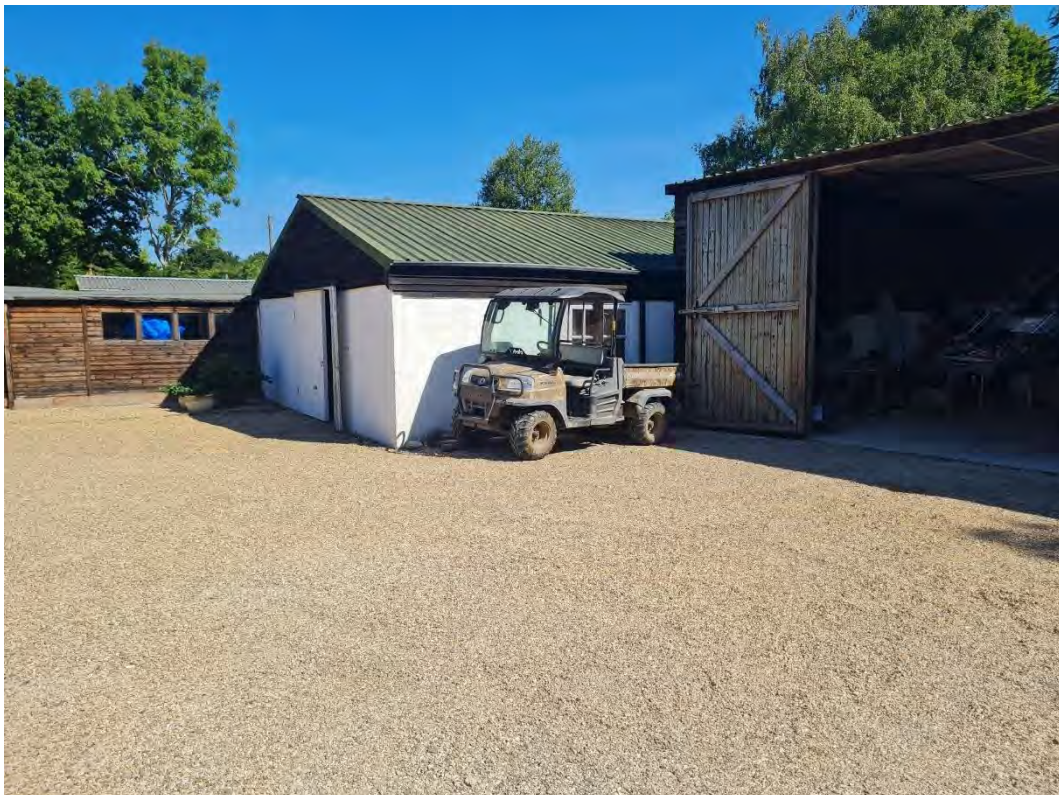
Front elevations of Buildings 1 & 2
