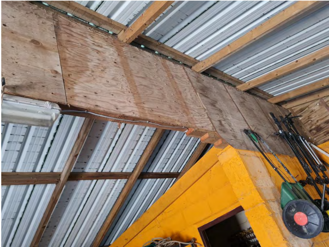
Internal view of Building 1 including equipment storage
