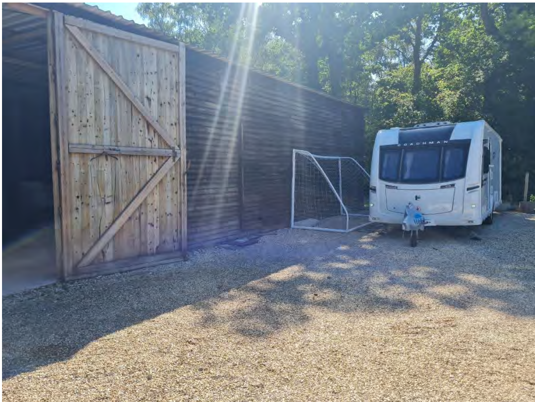
Front elevation of Building 2 and caravan parked adjacent
