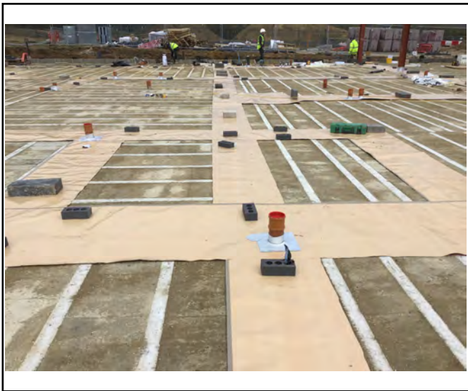
Membrane installation
