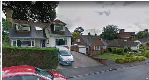
1 Kendal Close (raised eaves & dormer size and form)
