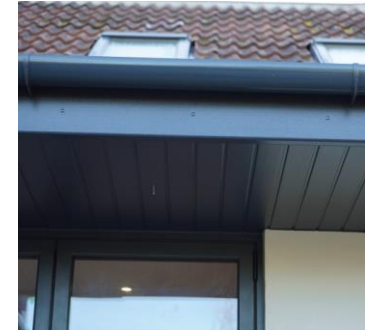
Black Fascias, Soffits and Rainwater Goods
