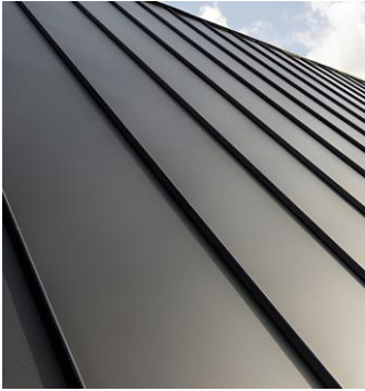
Standing Seam Roof for Rear Extension
