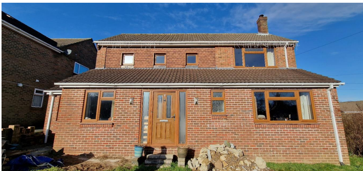
Picture 1: The front of the house showing the hanging tiles area and the front single storey extension, which were created 8 years ago.
