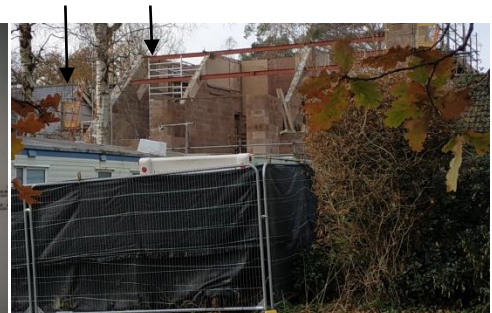
No.9 Under Construction (not at full apex height yet)
