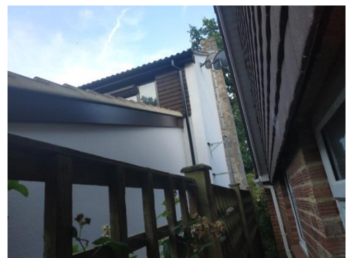
Gap viewed from rear
