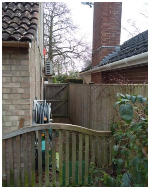
Gap viewed from rear
