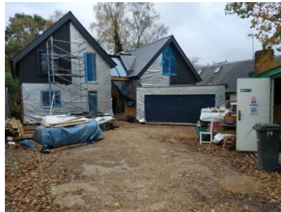
No.14 Under Construction
