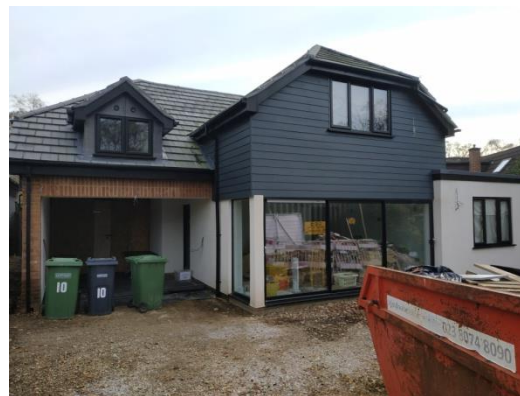
No.10 Under Construction
