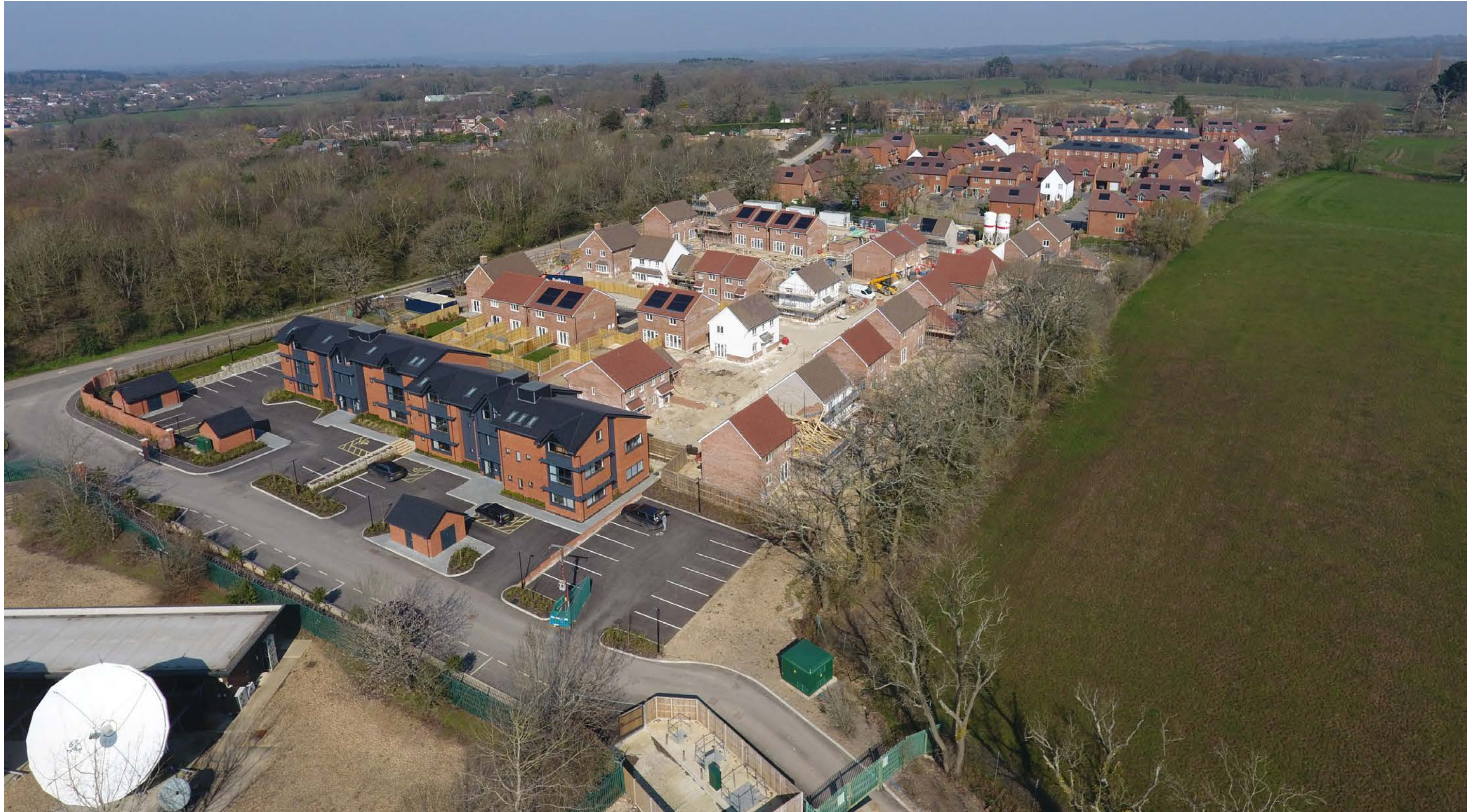
AERIAL VIEW OF EXISTING DEVELOPMENT AT KNOWLE LANE
