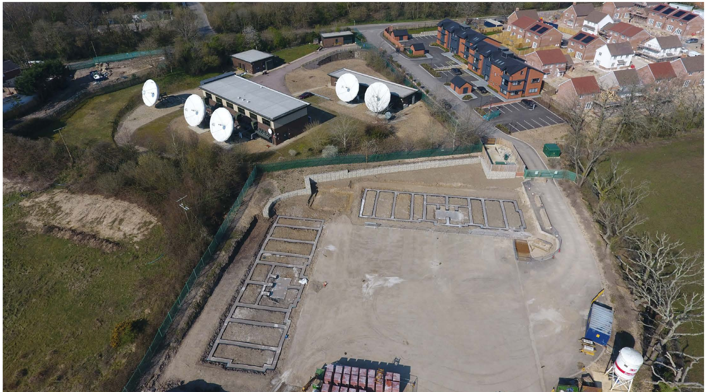
AERIAL VIEW OF EXISTING DEVELOPMENT AT KNOWLE LANE - BUILDINGS B AND C OF PREVIOUS APPROVAL SHOWN UNDER CONSTRUCTION
