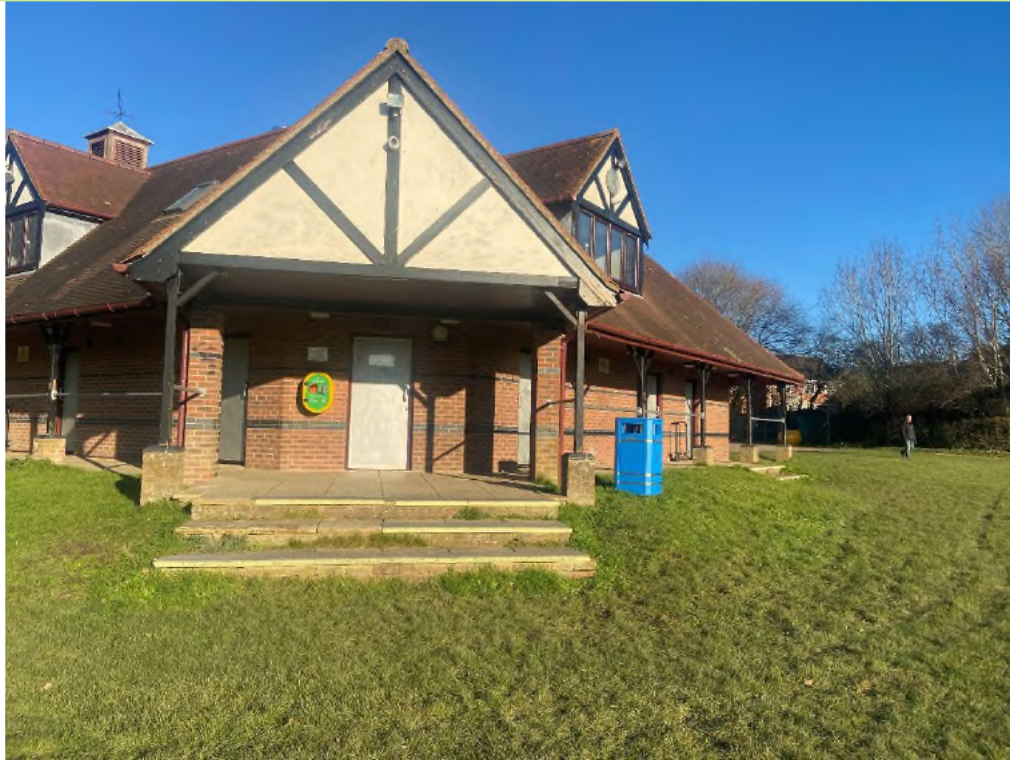
Plate 3 - Looking north east at Pavillion
