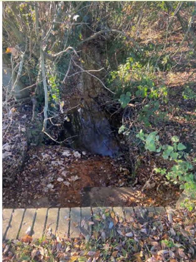
Plate 5 -Standing on culverted part of drain looking westward
