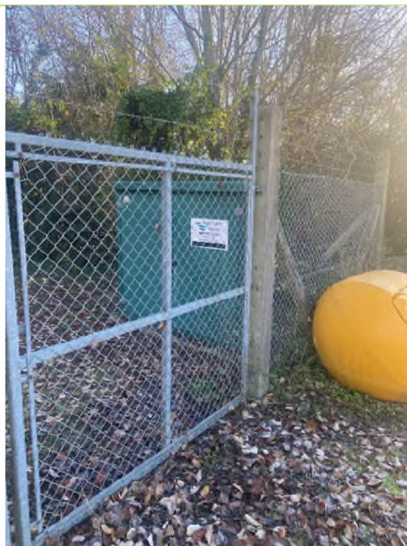
Plate 2 – Looking at Waste Water Pumping Station
