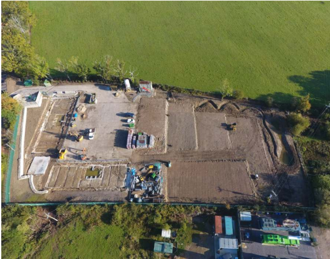
Figure 6: Recent aerial photograph of site
