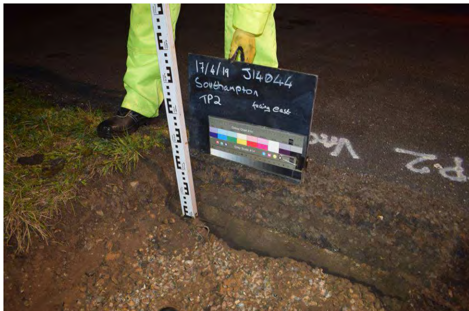
TP2 eastern face (runway edge)
