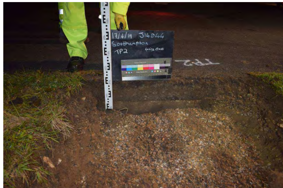
TP2 eastern face and de-lethalisation concrete
