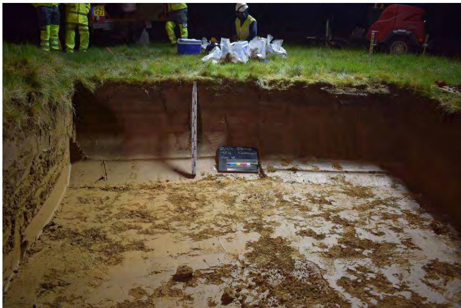
TP4 western face and base
