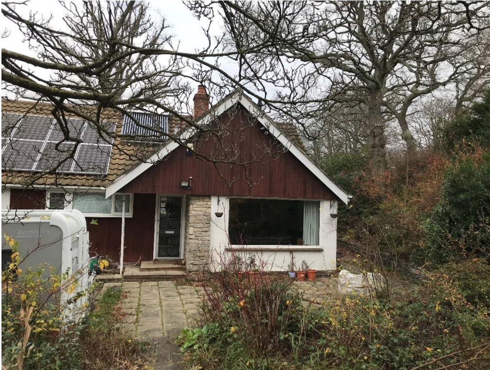
Existing entrance to dwelling, facing north
