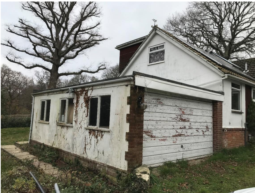
Existing garage to be demolished, facing northeast
