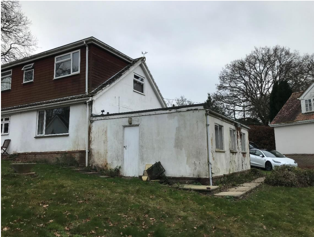
Rear (north) elevation of garage to be demolished
