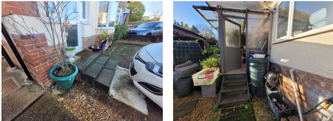
Figure 8 Views of property showing existing raised floor level
