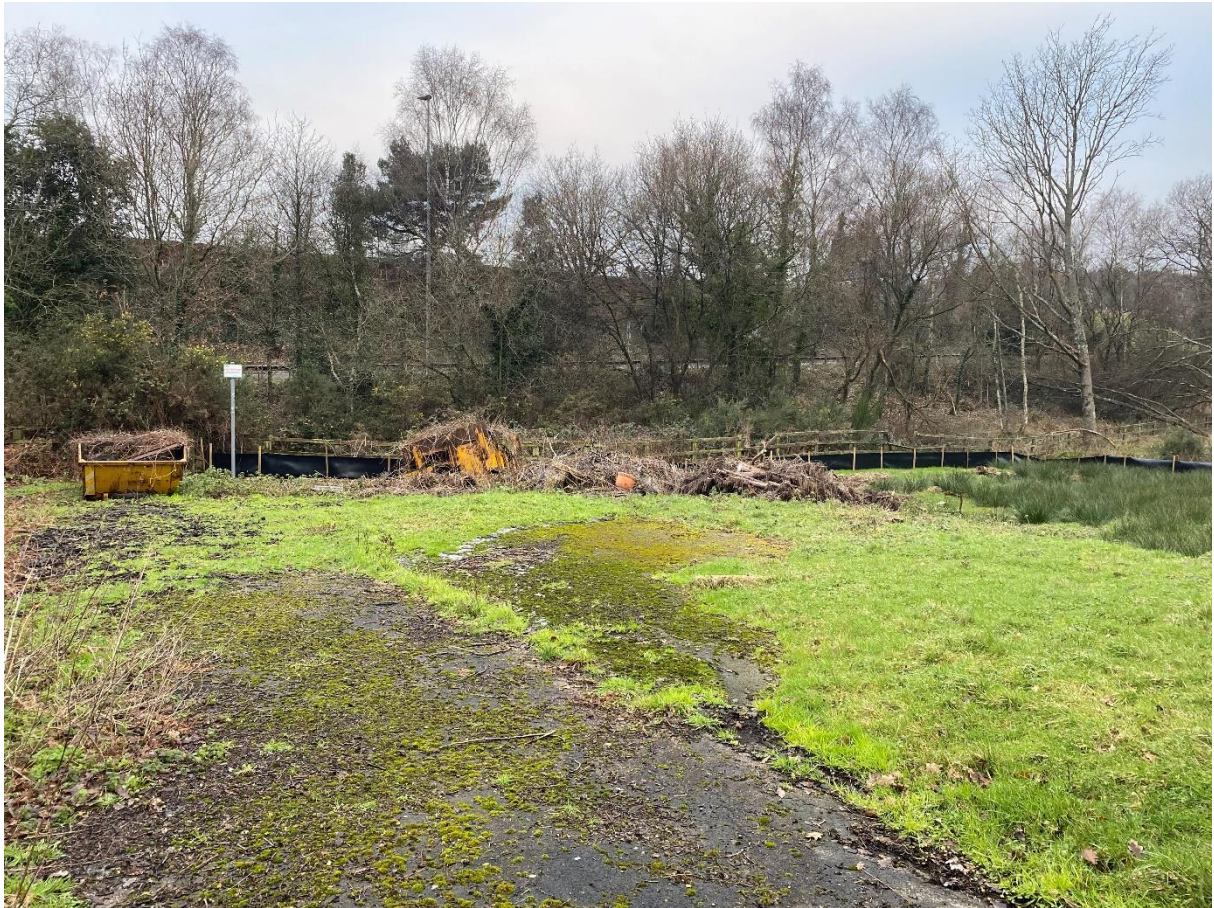
SAL5 Construction area looking to the west towards the M3 at top of the embankment. Tree protection barriers to be installed within 1m beyond the habitat / ecology fence.
