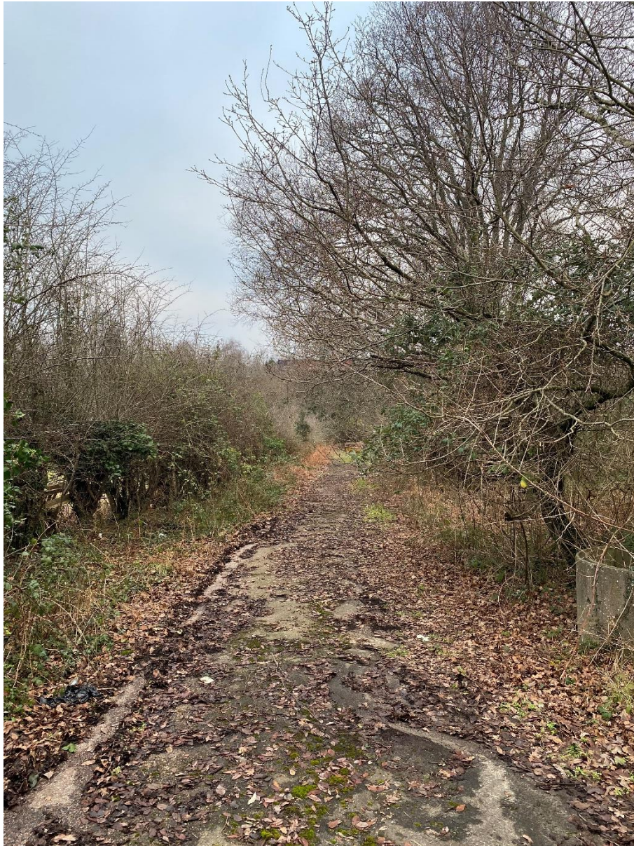
SAL2 Access road to site near turn into field to north. Tree works to 5m above asphalt and 1m offset from the asphalt necessary to allow construction access. Tree protective fencing to be installed either side of the access from this point forwards in to the site.
