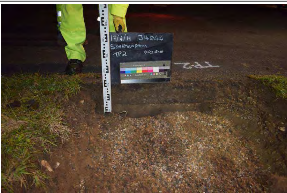
TP2 eastern face and de-lethalisation concrete
