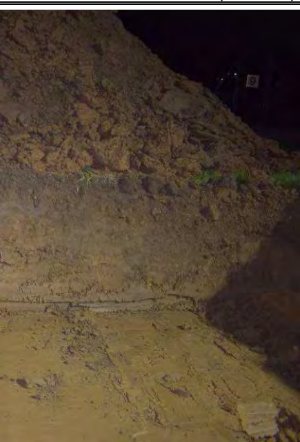
Topsoil and base
