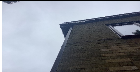
Photograph 9. Fascia and soffit north west of B1 20/02/23
