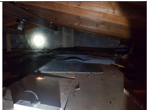
Photograph 6. The roof space of B1
