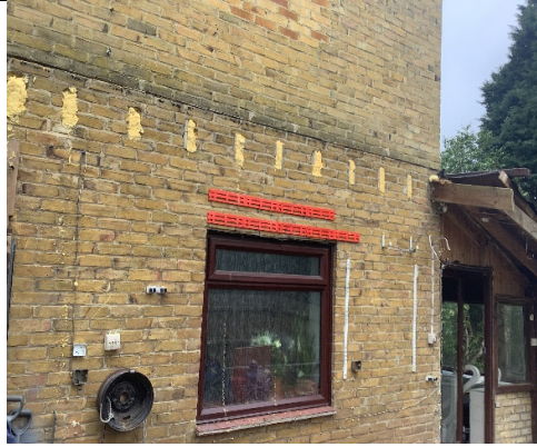
Photograph 7. Cavity wall east of B1 20/02/23
