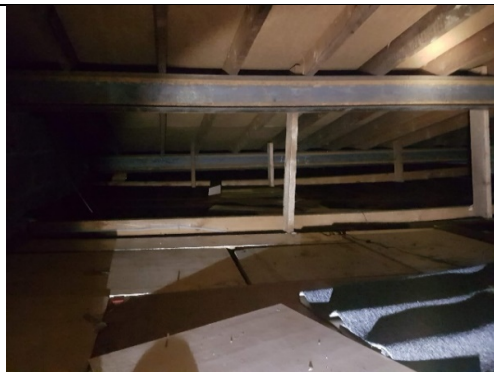
Photograph 5. The roof space of B1
