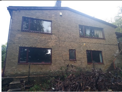
Photograph 1. B1, northwest elevation
