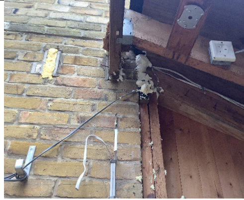
Photograph 8. Wooden Porch east of B1 20/02/23
