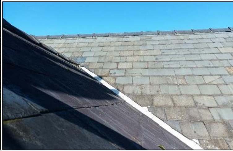
Figure 2 – northeast elevations roof structure and coverings (B1)
