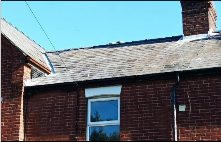
Figure 5 – southwest elevations roof
