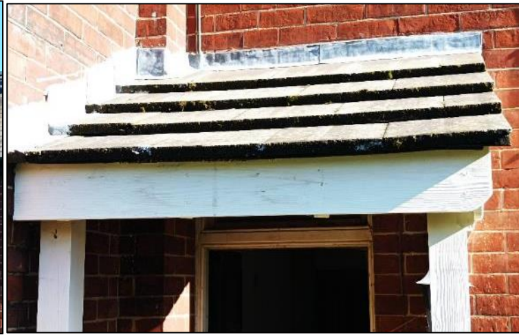
Figure 6 – porch entrance on southwest elevation
