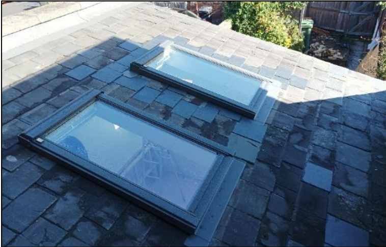
Figure 3 –northeast elevations lean-to extension
