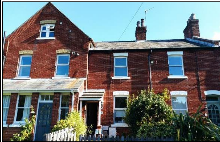
Figure 4 – southwest elevation of B1
