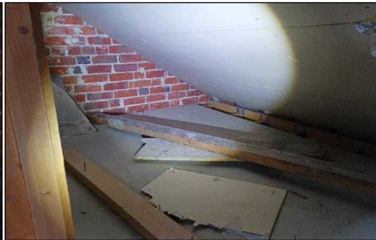
Figure 8 – eaves on southwest elevation
