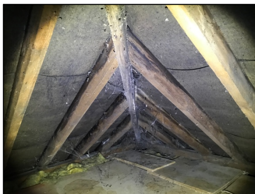
Figure 8 – roof void with lining and insulation
