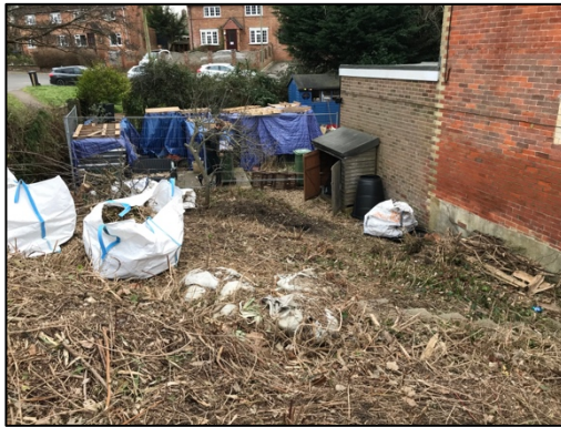
Figure 4 – cleared scrub area east of the dwelling
