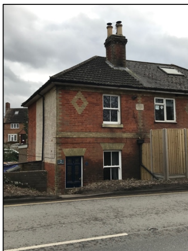
Figure 6 – northern house elevation with brick chimney
