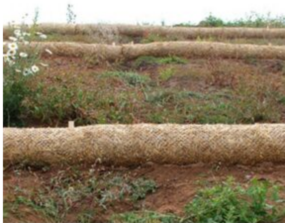
Example of Hy-Tex straw wattles on a working site
