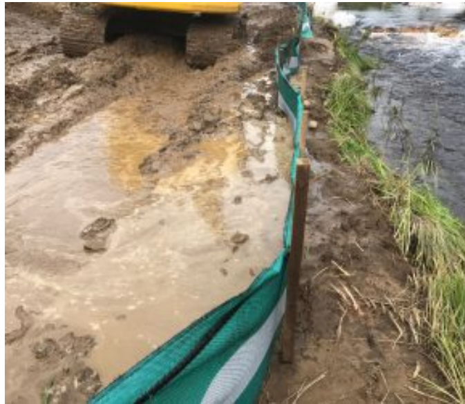
Example of Terrastop Premium on a working site
